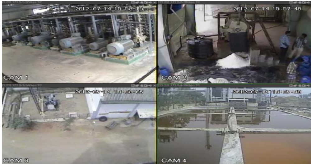
Fig. no. 6.14- Picture showing images of the CC cameras
