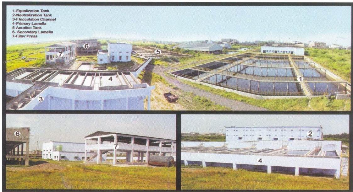
Fig. no. 6.12- Photographs of CETP of Sachin Infra Environment Ltd.
