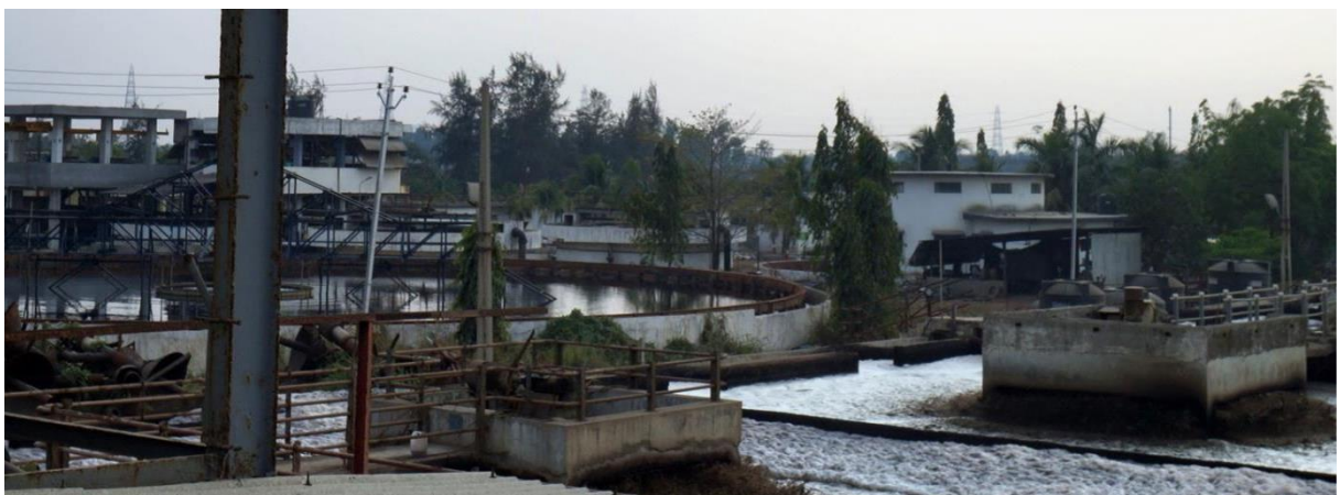
Fig. no. 6.21- Impression of the aeration tanks and the secondary clarifiers (March 2014)
