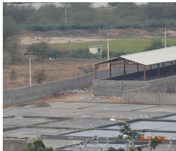
Solar Evaporation Pan
