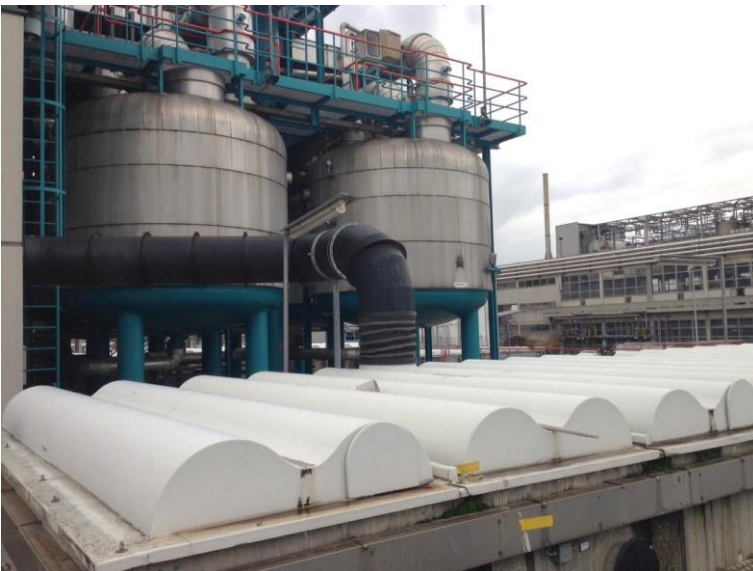
Fig. no. 6.20- Treatment train, aerial view and GAC adsorption for air pollution control at the CETP Basel (Source: ProRheno AG)
